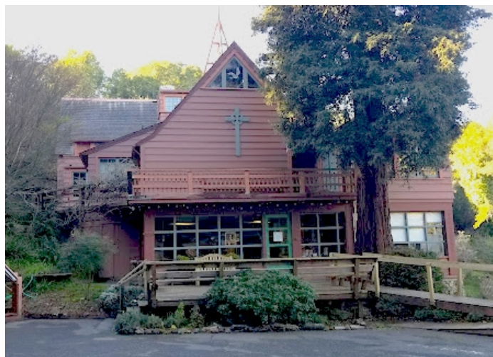
St. Columba Episcopal Church & Retreat House in Inverness
